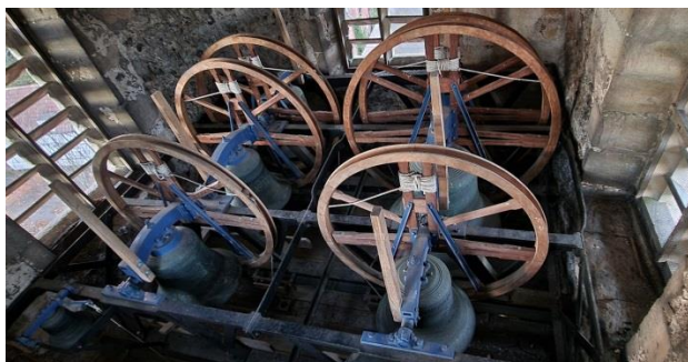
Bell Installation November 2022
